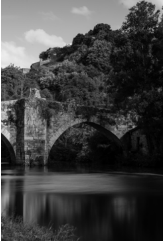
A Ponte de Vilanova and Alameda do Arnado
